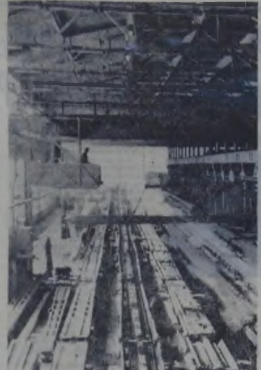
Sectia de stilpi precomprimati in Intreprinderii de prefabricate Roman
